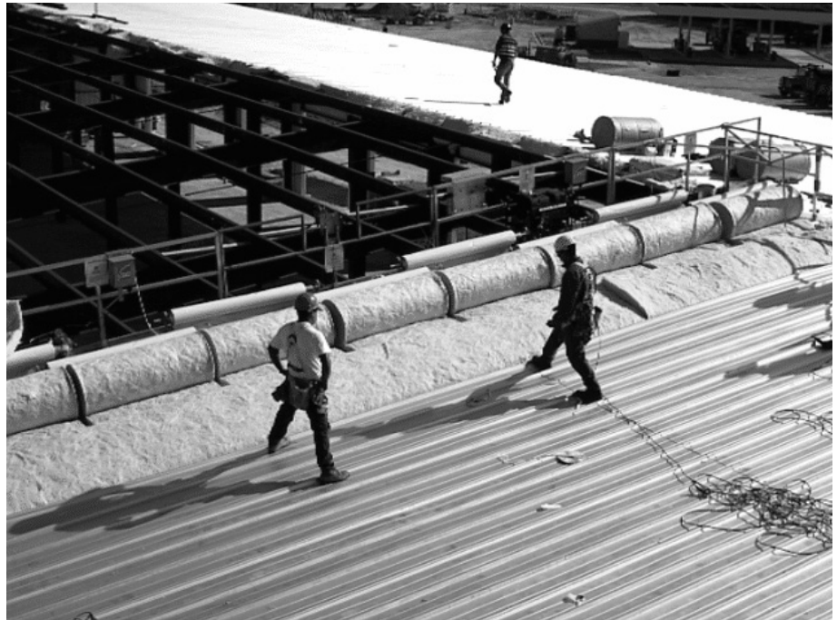
300 Series installing double layer.
