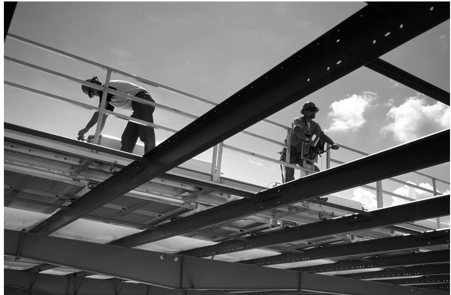
300 Series installing single layer.
