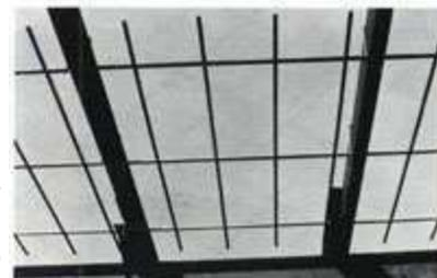
slide out from main frames and drop into position. *No fasteners or tools required, all work is done from the topside.*
